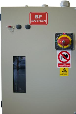
Inverter fully installed in a self contained cabinet with circuit breaker, ELR/GFI and internal cooling fans
